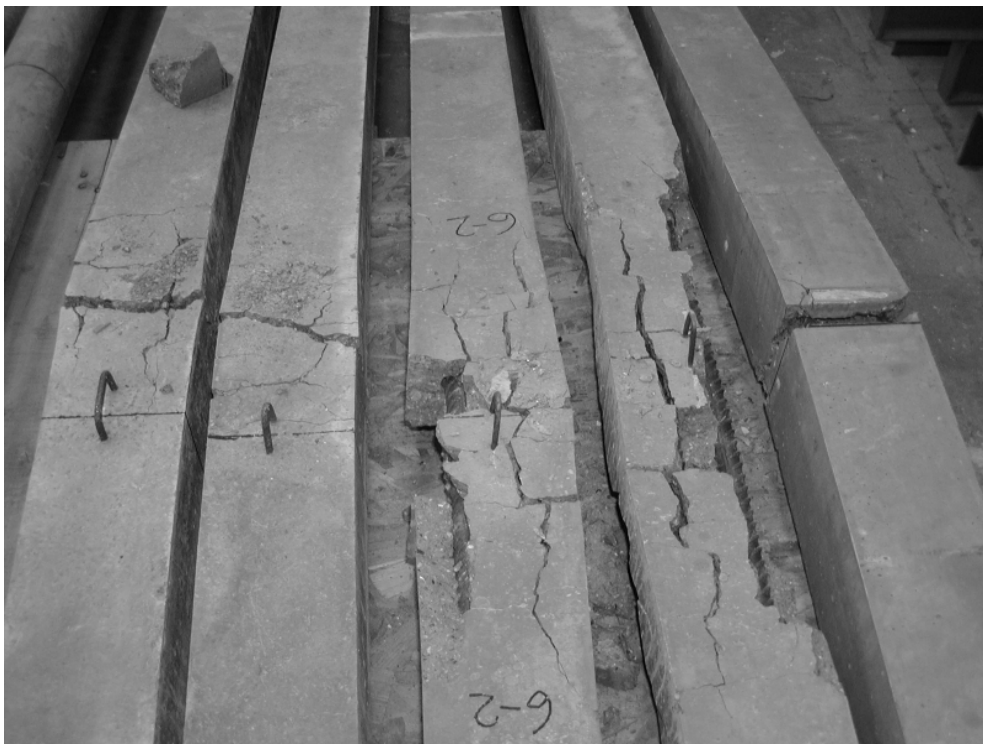
Figure 7 - Other columns tested at DTU. The one on the far right shows failure at a stirrup, while the centre column shows a cover to the reinforcement considerably larger than the nominal cover of 15 mm.
