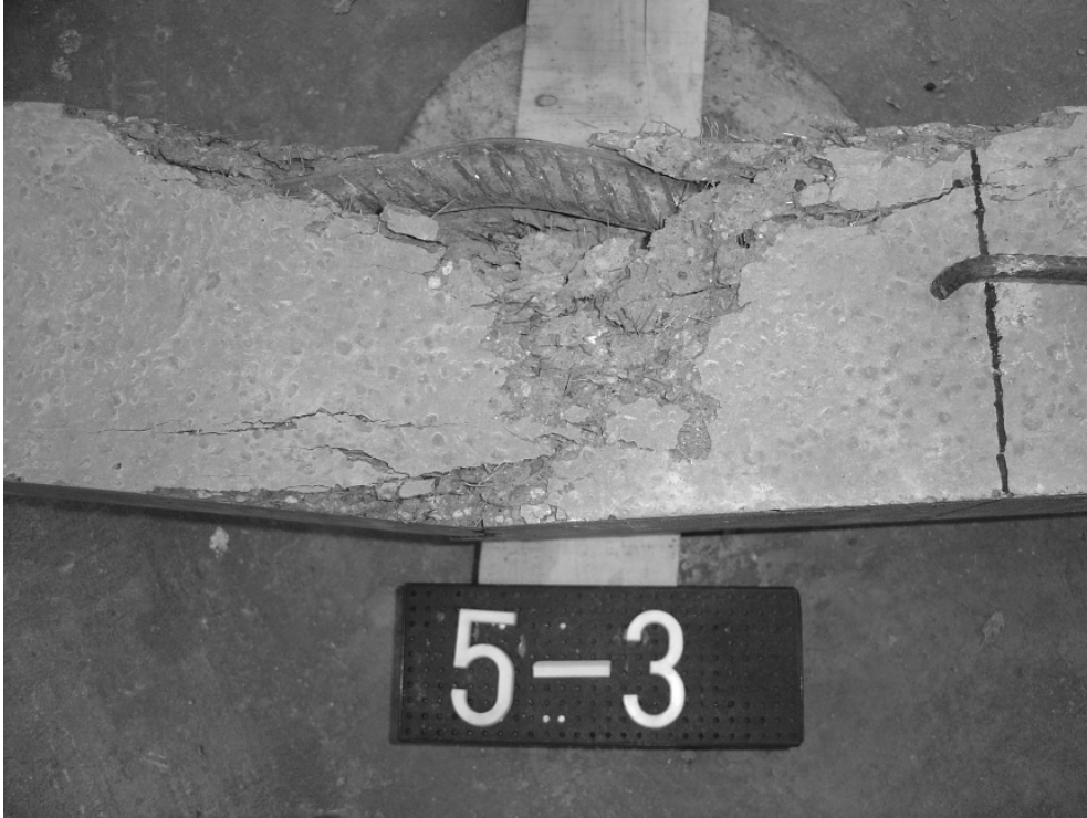
Figure 6 - Column tested at DTU with 120x120 mm cross-section, 2% fibres, length 3898 mm, reinforcement 4Y16, maximum test load 1430 kN.
