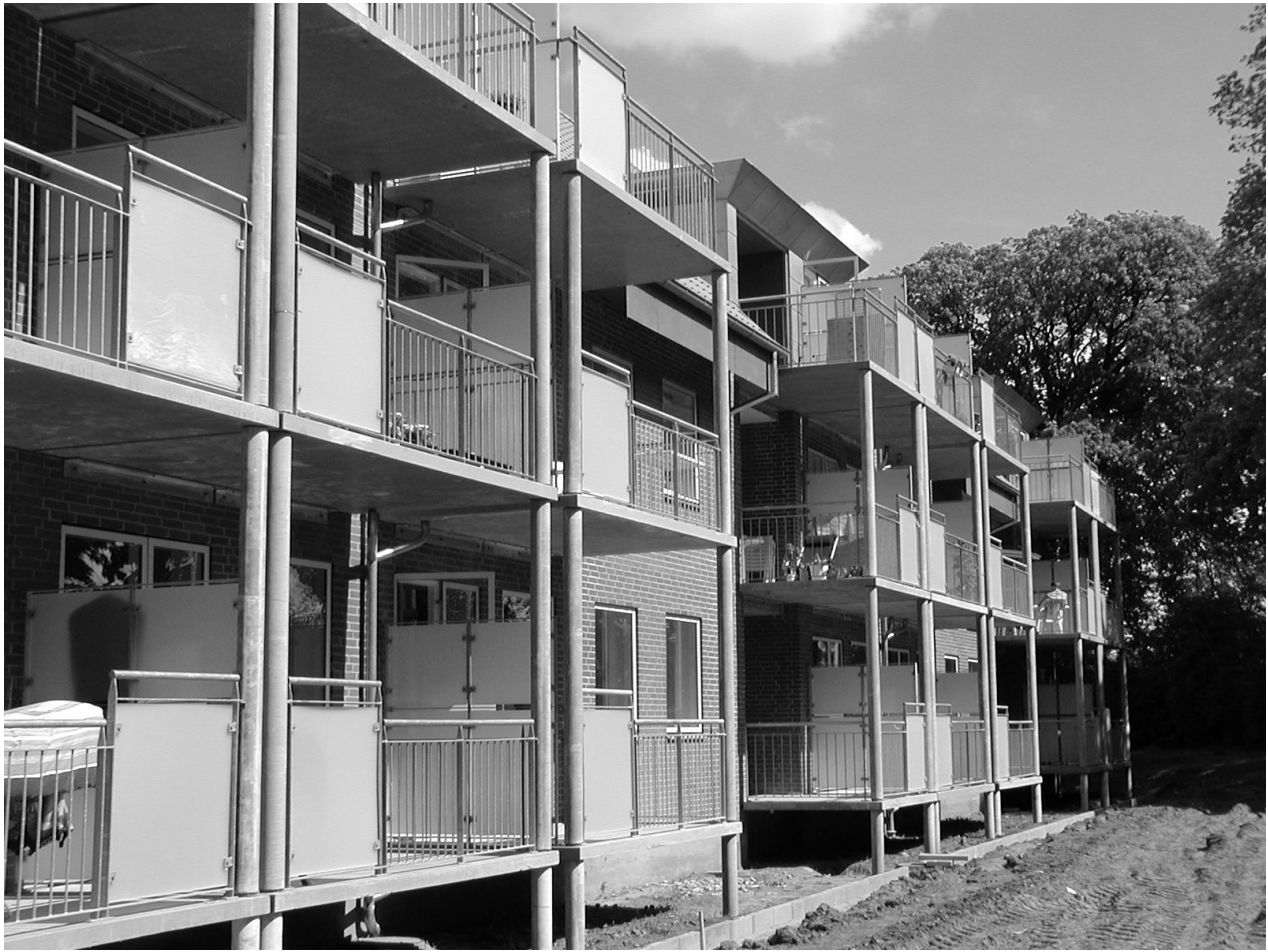
Figure 10 CRC Balcony slabs and columns produced by Hi-Con at Askehaven, Vejle in Denmark.
