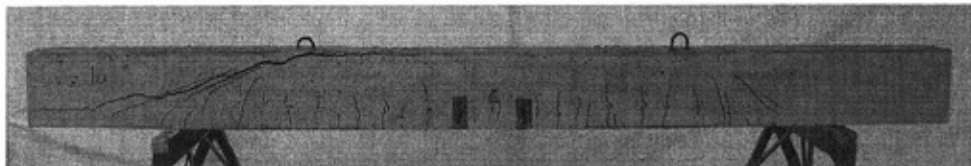
a) Crack pattern large beam S1.
