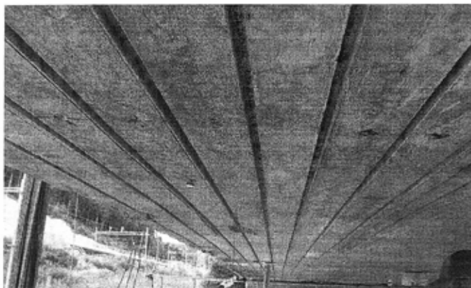
Figure 6 – Grooves were sawn in the bottom of the slab (15 x15 mm) and then filled with a resin and rods of CFRP (10 x 10 mm) in order to enhance the flexural resistance of the slab, [16], [17].
