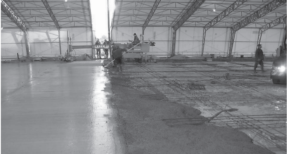
Figure 1 –Placing of concrete over the preinstalled reinforcement in strips was trough the tent roof. Here the last moments before power floating, placing of the hard concrete screed using a LASER ARM® laser screed machine and manually bull-floating the surface of screed (2).
