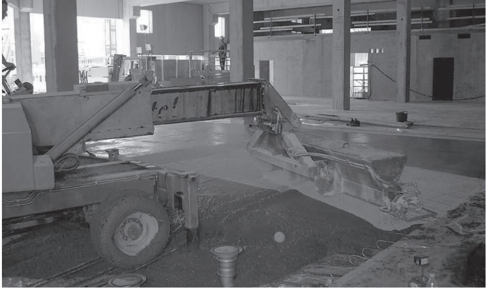
Figure 3 – Placing of the hard concrete screed using a LASER ARM laser screed machine in the narrow environment between precast concrete columns in this heavy building (9).
