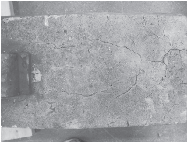
Figure 9 – Cracks at the end of a B63 sleeper [6].
