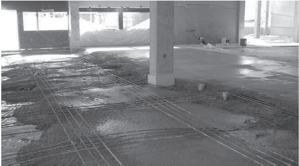
Figure 2 –The concrete is placed in layers due to its thickness 400 mm. It was windy inside due to uninstalled facade windows, but this fact did not seem to impair the quality in this case (9).
