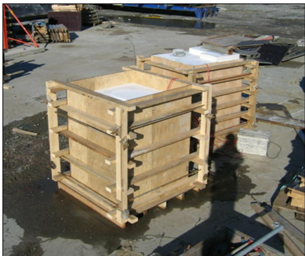
Figure 6 – On-site 1 m 3 semi-adiabatic calorimeters [5]
