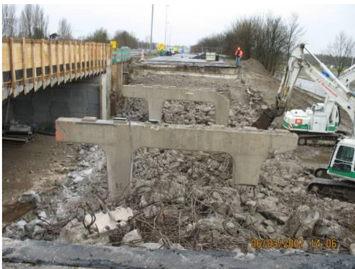
Figure 5 – Demolished concrete viaduct which suffered from deleterious ASR.
