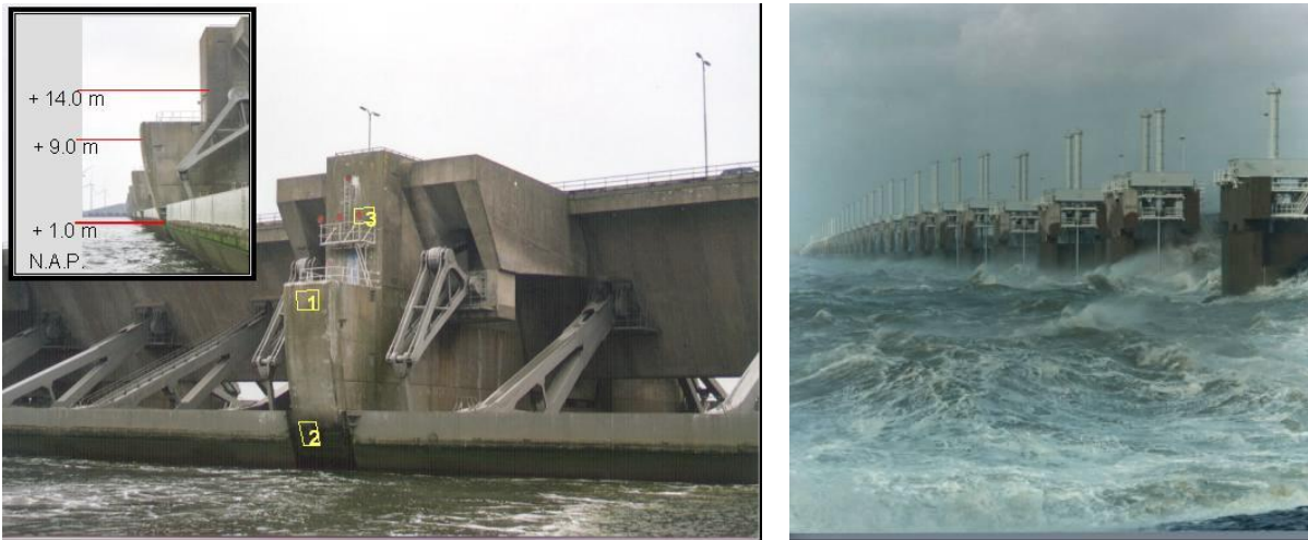
Figure 2 – Discharge sluices in the Haringvliet dam and Eastern Scheldt storm surge barrier.
