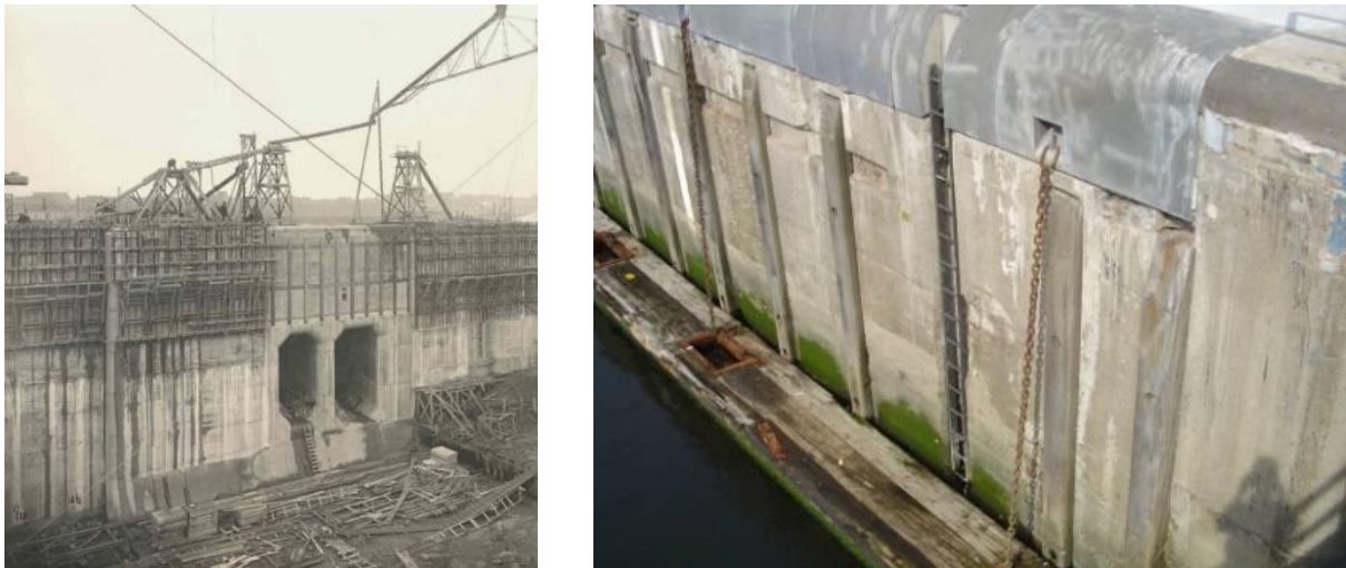
Figure 1 – Lock walls of the Noordersluis at IJmuiden during construction (1921-1929) and after 80 years of service.
