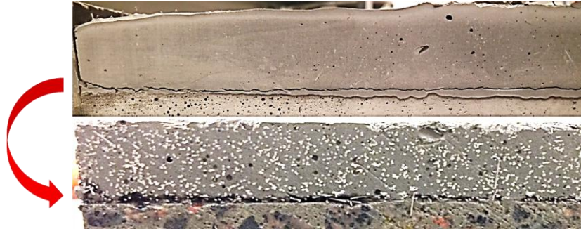
Figure 3 – An example of a severe delamination of the UHPFRC layer resulting in negligible bond strength.
