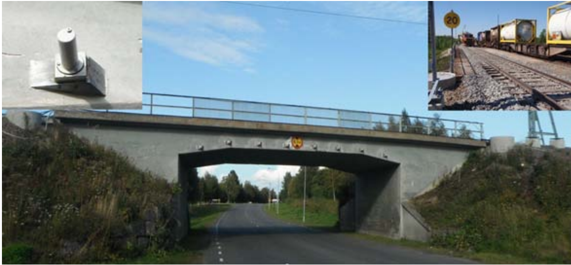
Figure 1. A concrete trough bridge built in 1959 in Haparanda close to the border to Finland. In 2012 the bridge was strengthened with eight post-stressed bars installed in holes drilled through the slab (insert left). In this way it was possible to increase the bending and shear capacity of the slab to enable an upgrading of the line from an axle load of 25 to 30 ton (insert right shows traffic on the two tracks on the top of bridge), see further MAINLINE (2014).
