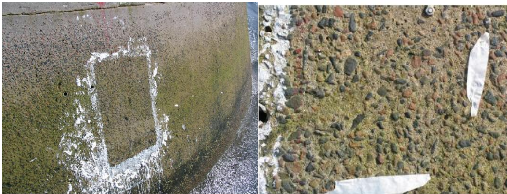
Figure 1 - 0.3 mm/year concrete ice abrasion on 90 MPa concrete of the Canadian Confederation Bridge, left: pier, right: \sim 15 \times 10 cm close-up /Newhook 2007/.
