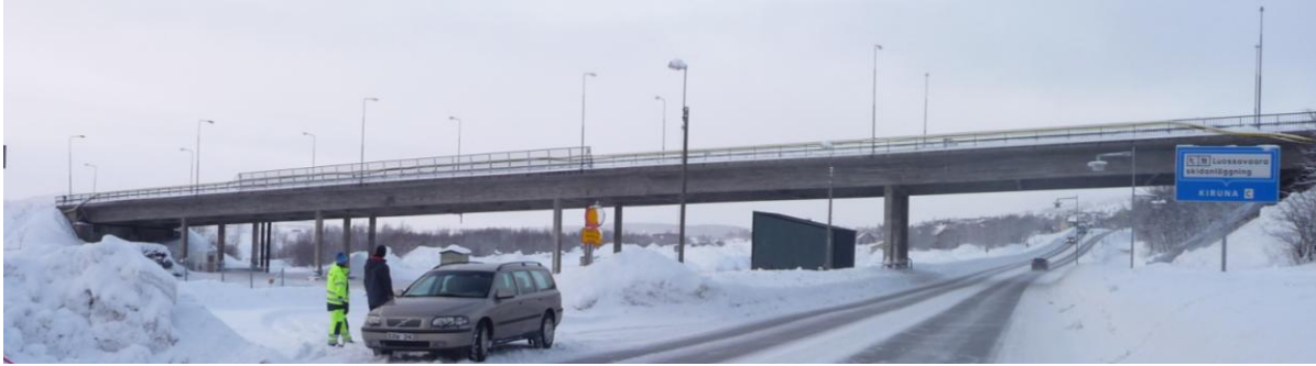
Figure 1. Photograph of the Kiruna Bridge, view from south (2014-02-19).
