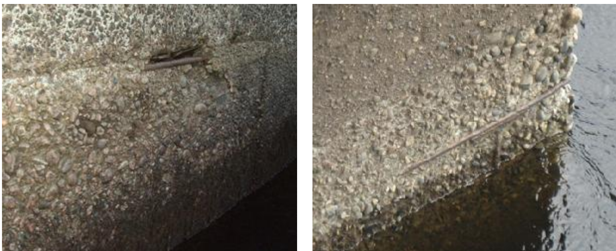
Figure 1 – Exposure of coarse aggregate and reinforcing steel at the waterline.
