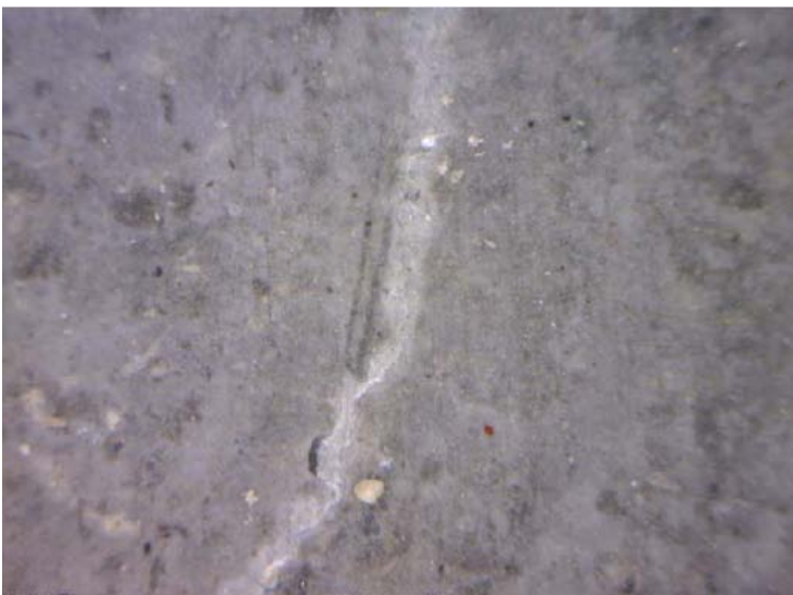
Figure 4. Photo of former cracks in concrete of EMC Cement, taken 5 months after formation in February 2013. The photograph shows that the former cracks have undergone a complete self-healing process without any intervention. During the observation period, continuous strength-development was also recorded by virtue of the ongoing pozzolanic reaction.
