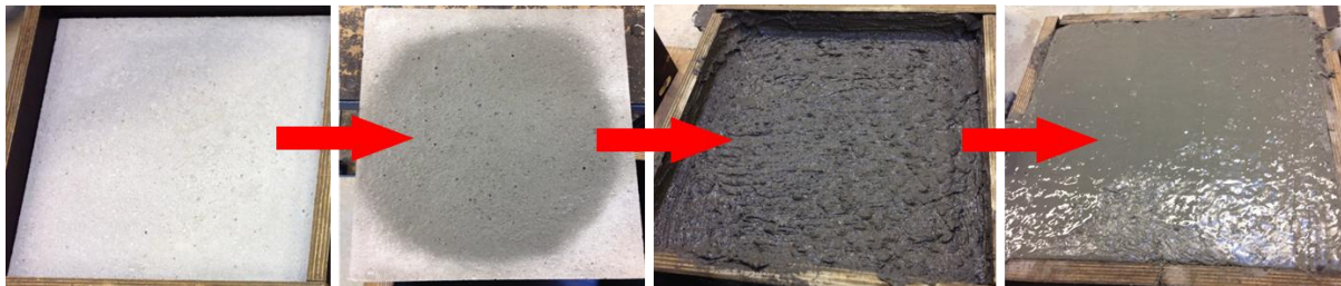
Figure 4 – A proper treatment of the substrate concrete before casting. The concrete surface was sand blast, moistened, and “penetrated” by a mortar bonding agent.
