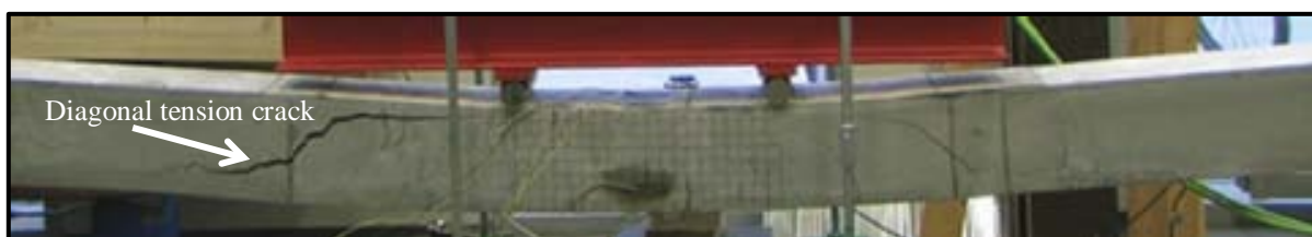
Figure 4 – Cracking behaviour for the test beam at failure (Gunnarsson, 2013).
