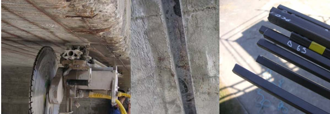
Figure 2. Near Surface Mounted Reinforcement, NSMR, can be placed in groves that are grinded in e.g. the bottom of a slab (left, middle). Carbon Fibre Reinforced Polymer (CFRP) bars (right) can then be glued into the groves, see e.g. Sustainable Bridges (2007), Täljsten et al (2011), MAINLINE (2014).
