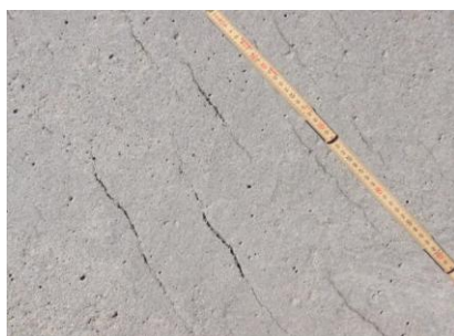
Figure 8 – Diagonal plastic shrinkage cracks in full scale observations
