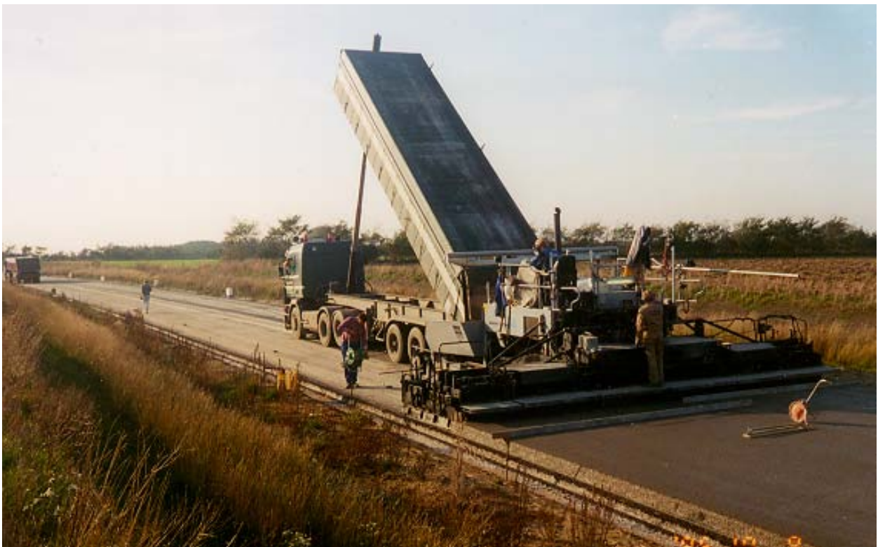
Figure 22: Concrete paving on the Hjørring ECOPAVE section
