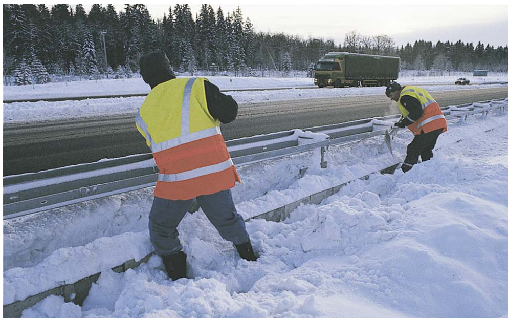
Figure 1 – The field exposure site at the highway R40 between Borås and Gothenburg
