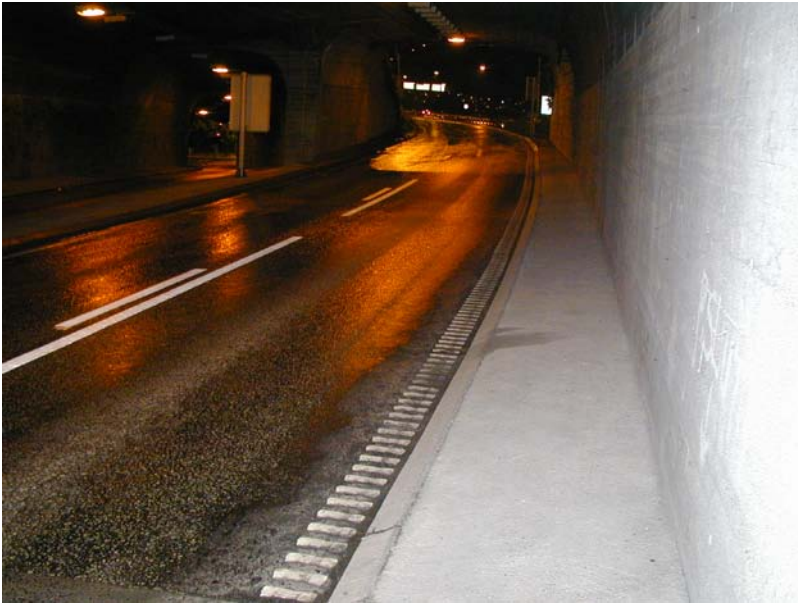
Figure 5: Bergen – Damsgård tunnel, Drilling of cores September 2001
