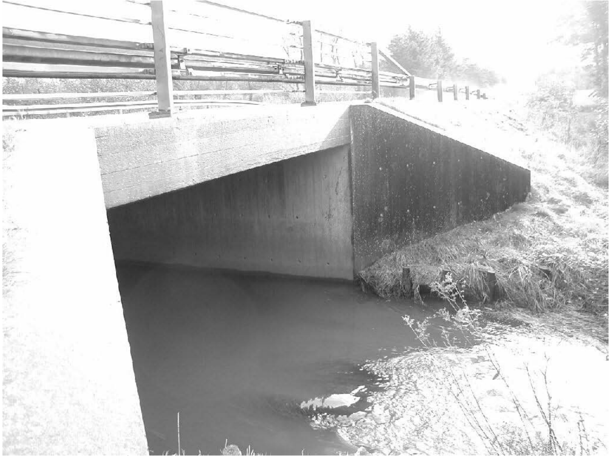
Figure 8 : Madum Å Bridge (Photo: November 2001)
