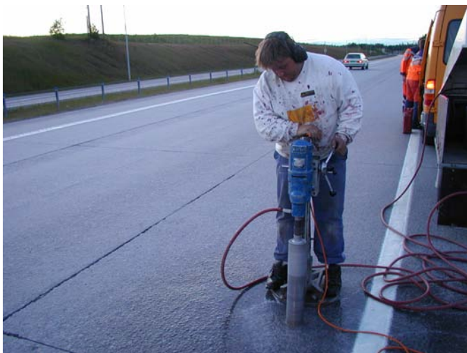
Figure 4: Akershus – Jessheim E 6, Drilling of cores June 2001
