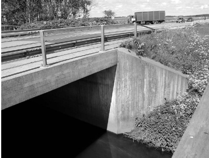
Figure 4: Sideview of the bridge
