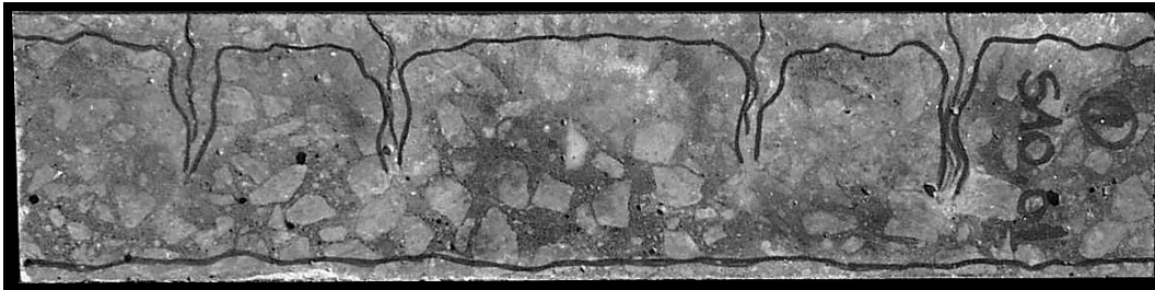
Figure 3 - Chloride exposed specimen after UV-test. Concrete SA-0. Exposure time 13 months. Load level 2.0 kNm. The beam contains 4 mechanically induced cracks, crack width between 0.21 and 0.32 mm. Overall average crack width 0.27 mm. Beam size in vertical direction 100 mm. Added lines: see Figure 2.
