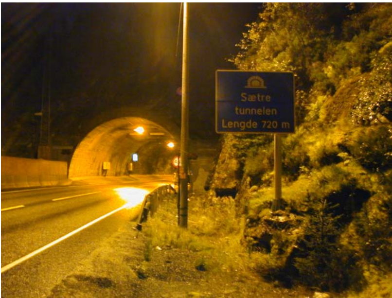
Figure 6: Bergen – Sætre tunnel, Drilling of cores September 2001
