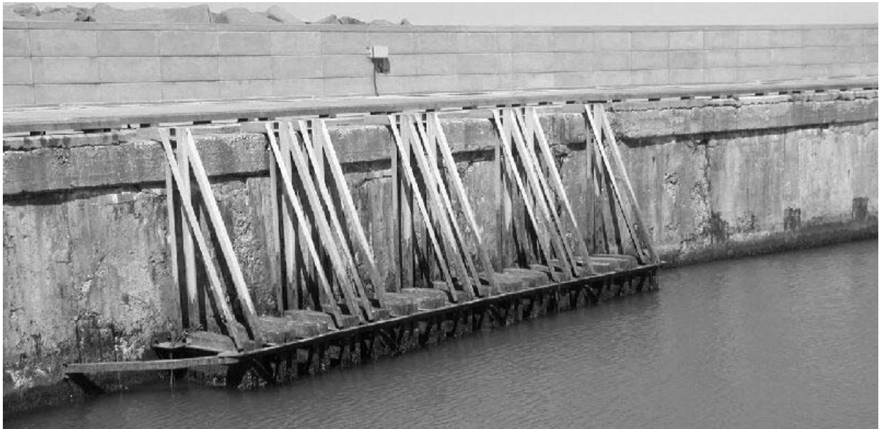
Figure 2B. Elements in Hirtshals Harbour, ebb tide. (Photographed in July 2001)
