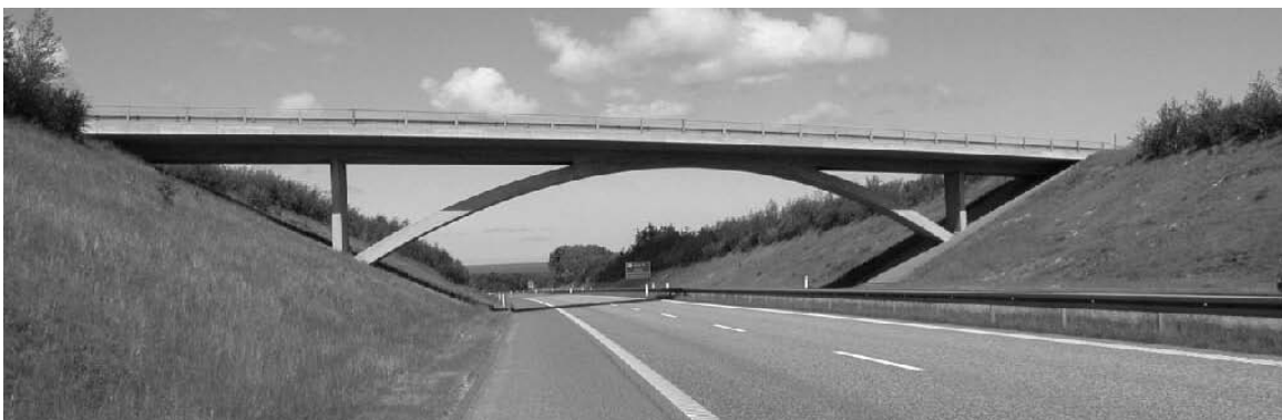
Figure 24: The high-strength concrete bridge, “Gadholtvej Bridge”
