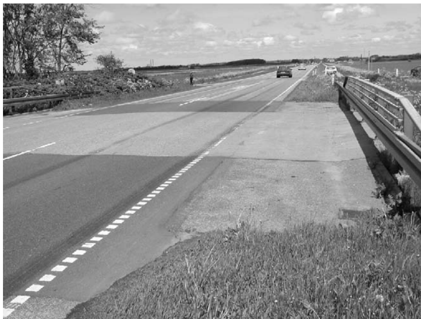
Figure 3: Photo of the Ryå bridge (July 2001)
