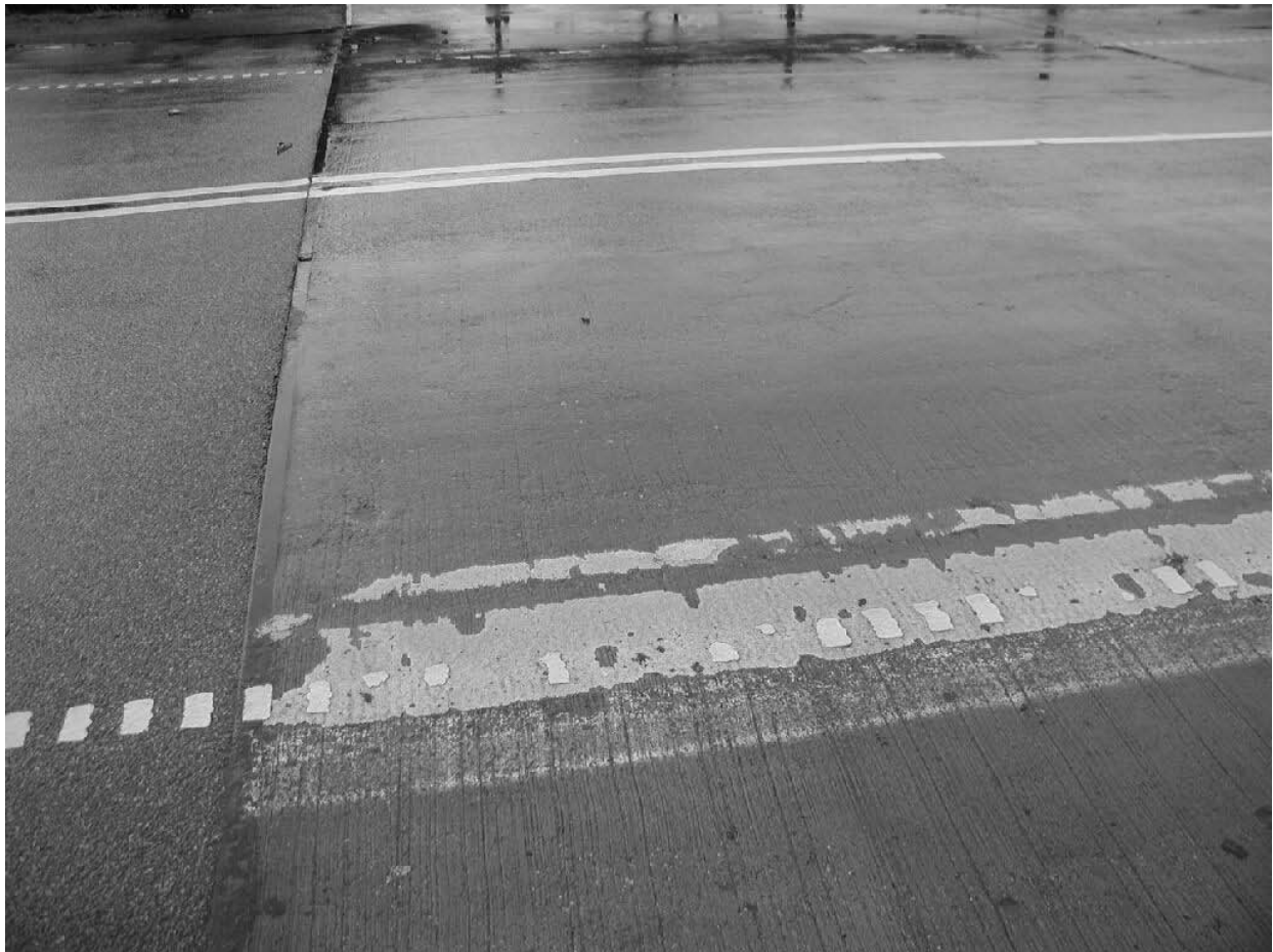
Figure 9: Surface of Madum Å bridge deck, November 2001
