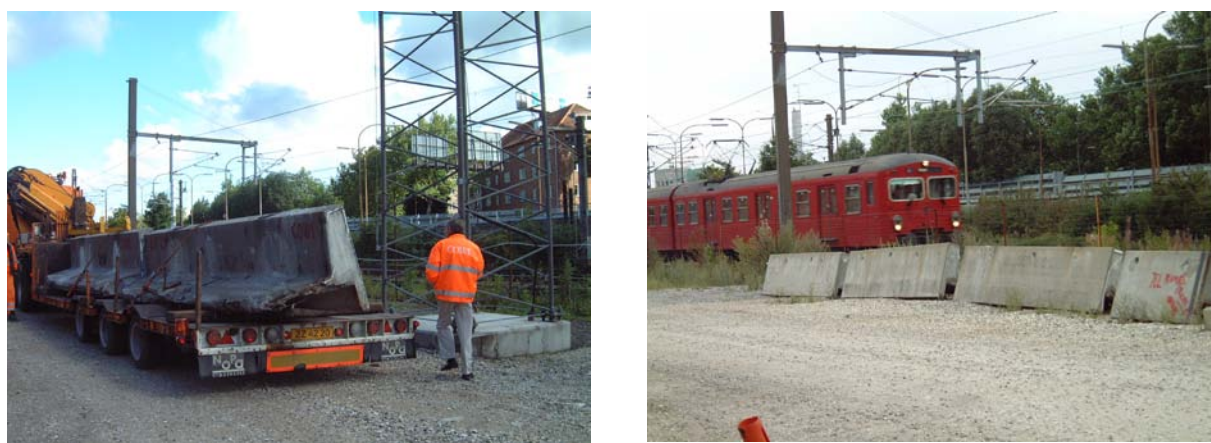
Figure 2 - Eight experimental edge beam elements from the Fiskebæk bridges are still kept for further studies.
