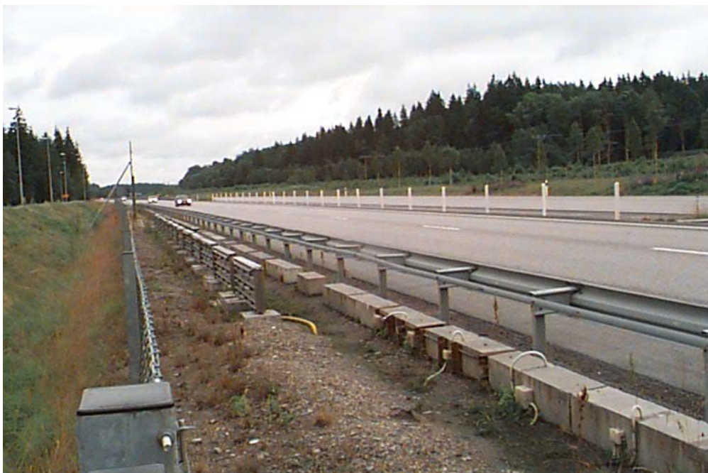
Figure 4 – The Rv40 field station. Concrete blocks placed along the highway Rv40.
