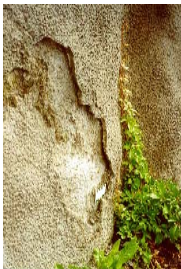
Figure 4 – Spalling after less than 13 years in a 1987 steel fibre reinforced concrete (SRPC and SF), due to TSA and carbonation due to PCD. A previous spray had been severely affected and was replaced after 17 years in service. Alum Shale environment, Åkebergveien Oslo.
