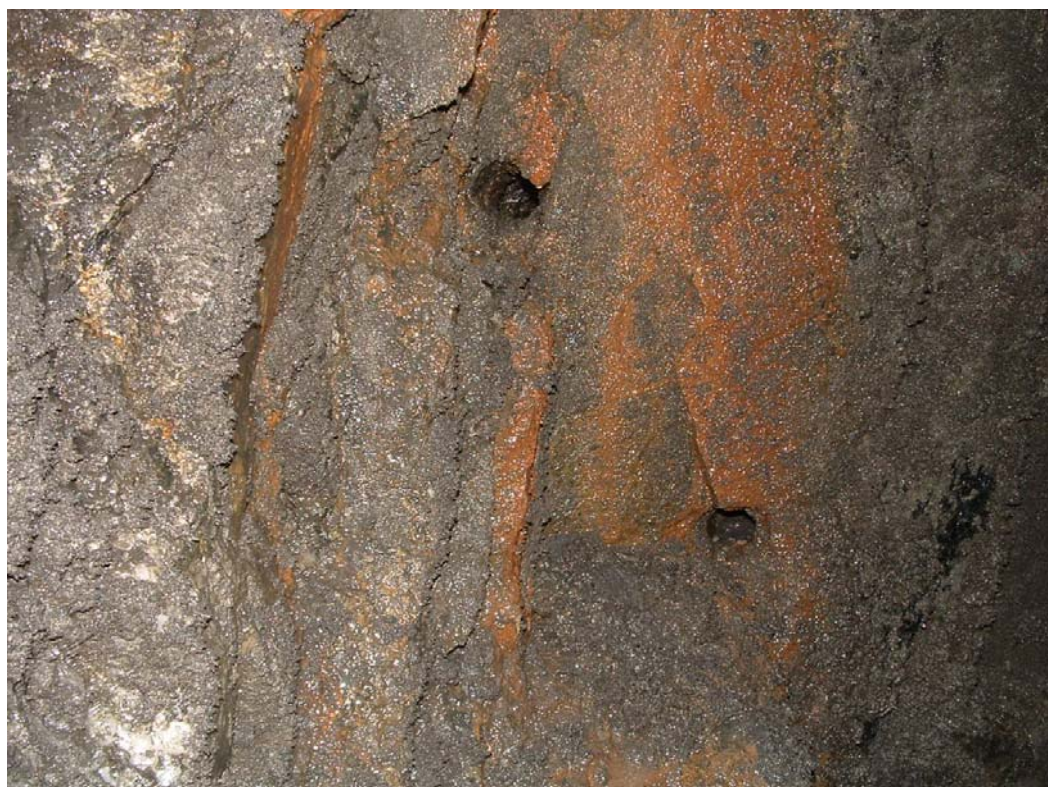
Figure 6 – Old core locations in the Freifjord subsea tunnel showing extensive breakdown of the sprayed concrete 16 years later. Rusty and black areas (right) consist of iron oxyhydroxides from Gallionella ferruginea and manganese oxides derived from Leptothrix sp. Grey deposits consist of gypsum formed from Ca in concrete and sulfate from seawater.
