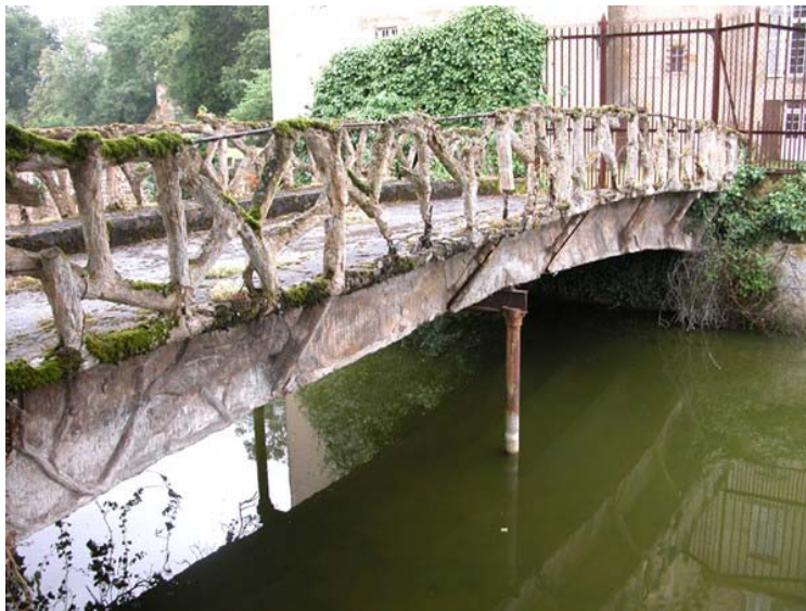
Figure 2 – Bridge at the Castle of Chazelet. Designed and built by J. Monier in 1875 with reinforced concrete
