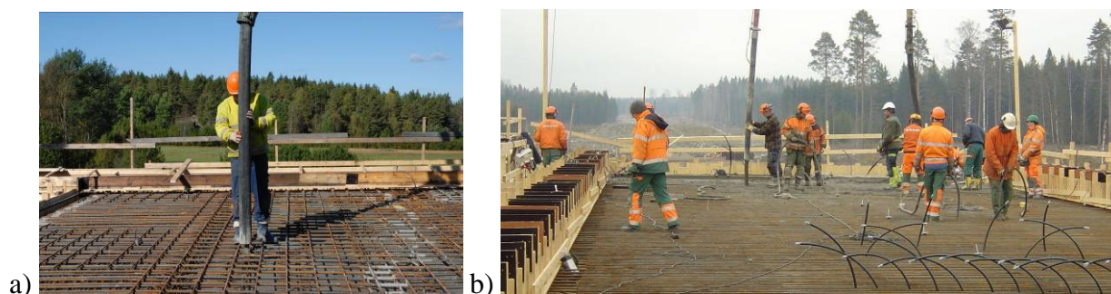
Figure 10: a) Casting SCC on the Nynäsvägen project. b) Casting of normal vibrated concrete.
