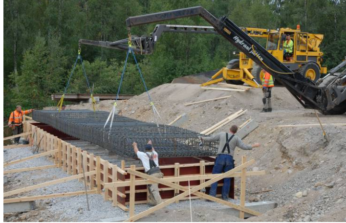
Figure 11: a) Normal working position for traditional placing of reinforcement. b) Cages of reinforcement placed directly in the form at the Kalix project.
