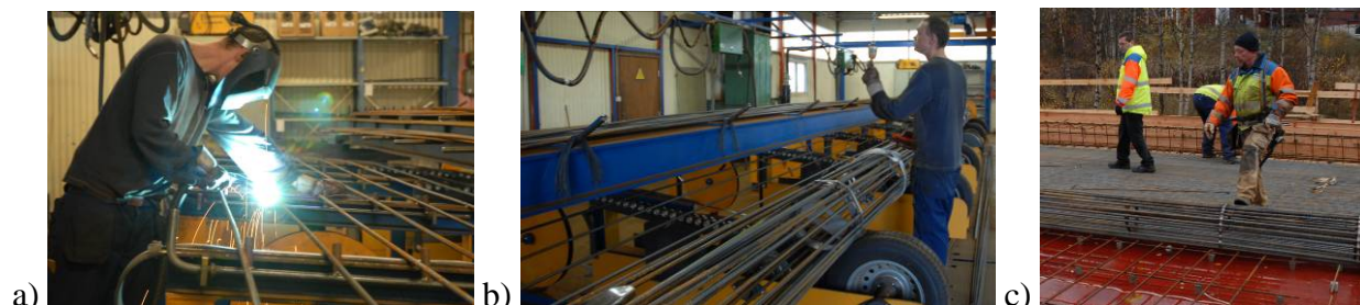
Figure 4: a) and b) Manufacturing of carpet reinforcement in a controlled factory environment. c) Placing of carpet reinforcement on the superstructure.
