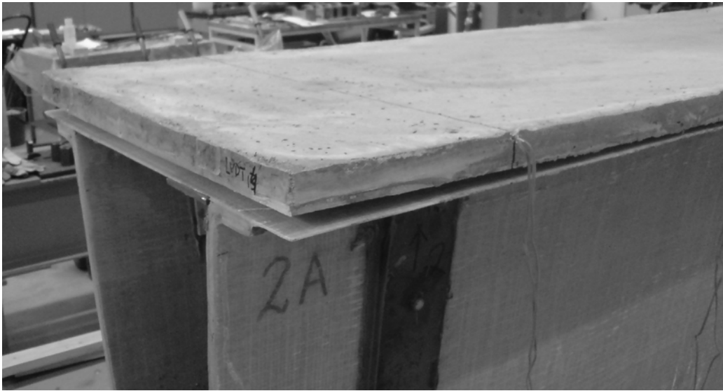
Figure 9. The test beam after loading to failure.
