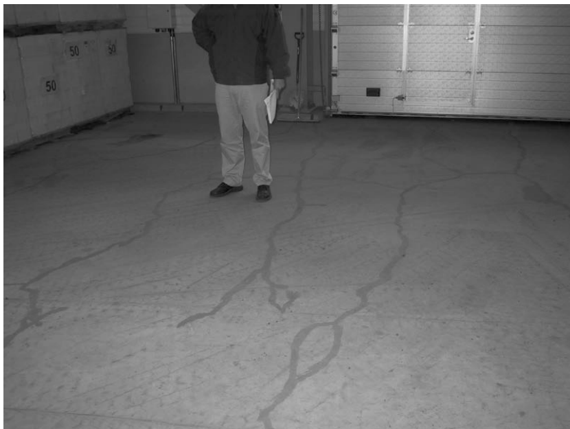
Figure 5. In many cases wide visible cracks has been filled up with epoxy. Most of the cases fissures were still able to detect after repairs.
