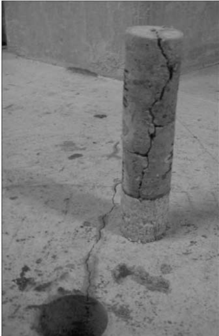
Figure 7. A drilled sample of a cracked slab.
