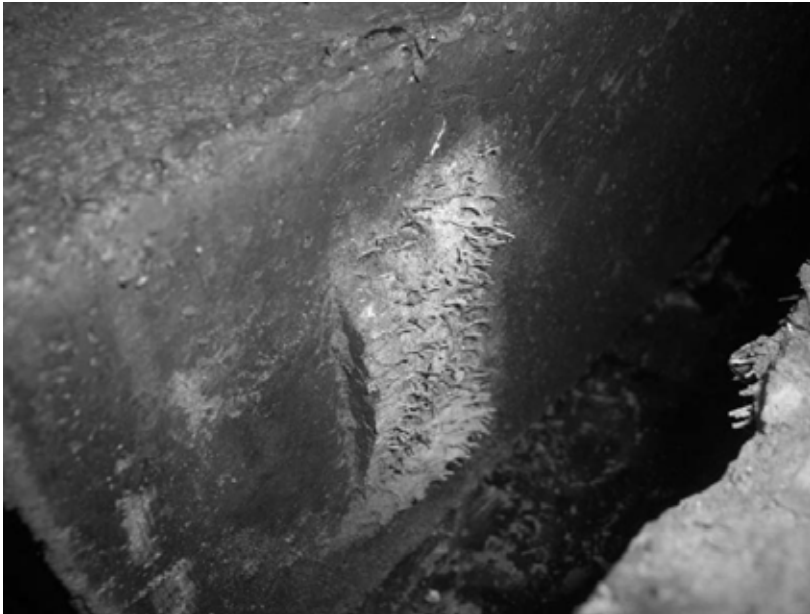
Figure 9 – Shear failure at indentation in joint detail 5, test no. 5.1, CRC JointCast, straight reinforcement with 40 mm overlap, three indentations 90 x 40 mm
