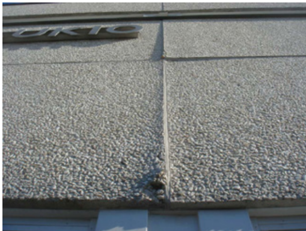
Figure 2 – Far advanced frost attack curves the edges of the facade panel.
