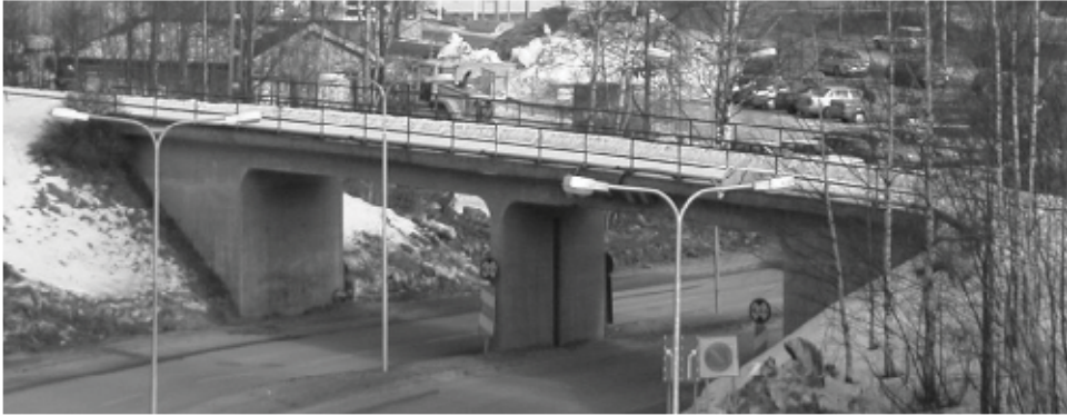
Figure 1 – The tested railway bridge in Örnköldsvik, Sweden.
