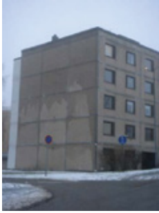
Figure 8 – Head of the concrete building in the beginning of a rain event. The upper parts get more rain than the lower ones.
