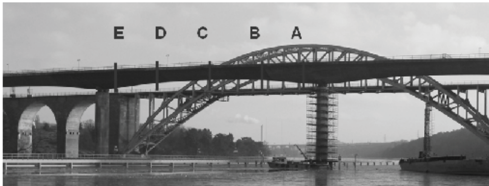
Figure 5 – Sections for monitoring of deformations in span P8 to P9.
