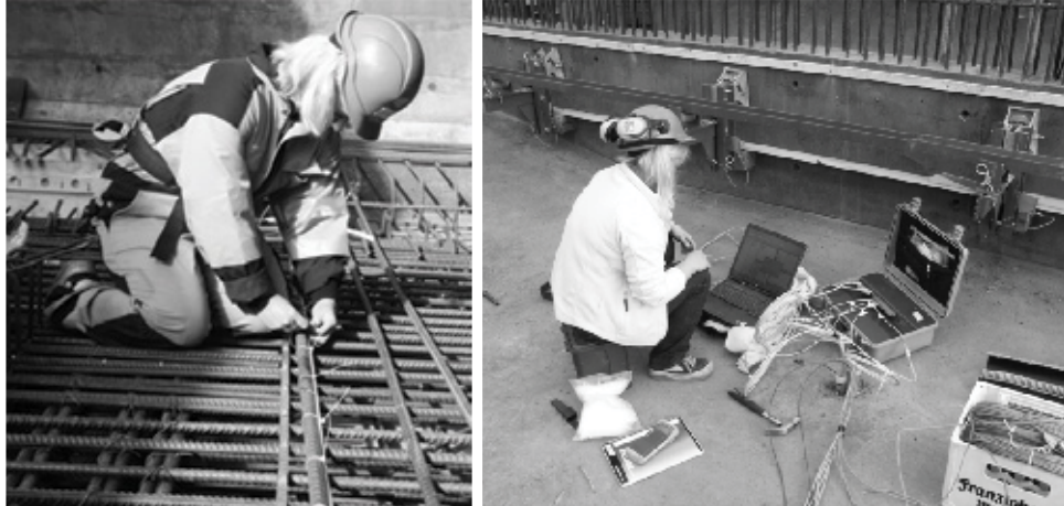
Figure 6 - Installation of a SOFO LG sensor on the rebar to the left and testing of sensors after casting to the right
