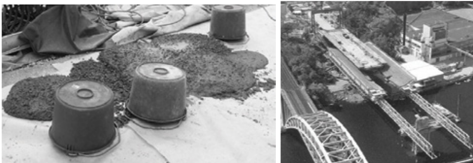
Figure 3 - Left: Concrete workability was tested on site for every concrete batch arriving on the lorries. Right: Also the formwork is red coloured.
