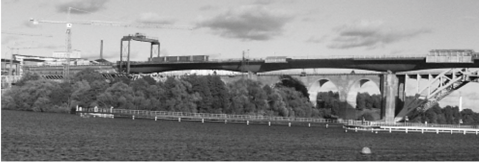
Figure 1- New Årsta Bridge during construction with the Old Årsta Railway Bridge seen in the background
