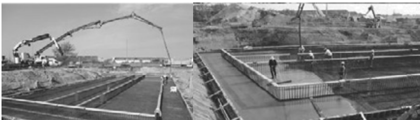
Figure 1 – Construction of the foundation slab cast with SFRSCC.
