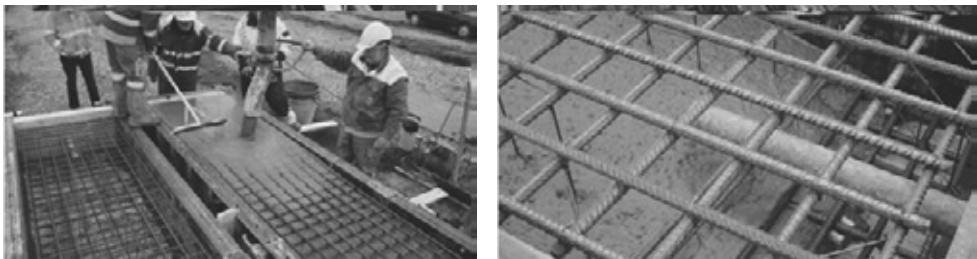
Figure 3 – Casting of full scale beam with SCC. Conventional reinforcement solution.
