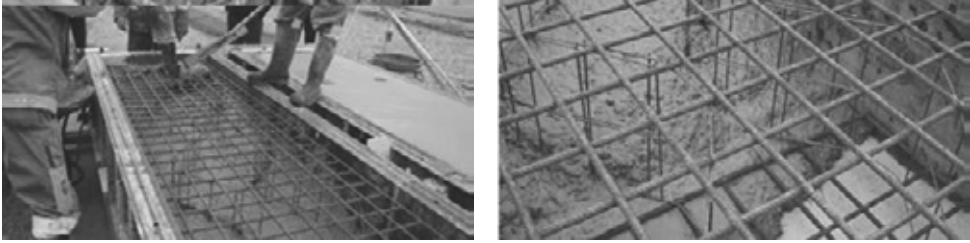
Figure 4 – Casting of full scale beam with SFRSCC. Combined reinforcement solution.
