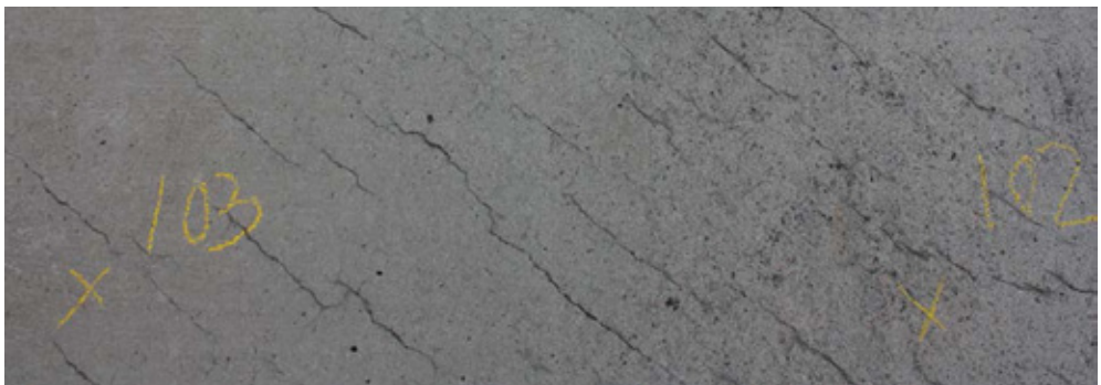
Figure 13 – North side of bridge A at mid-span. Macroscopic crack pattern mainly oriented 40-50° relative to its longitudinal direction.
