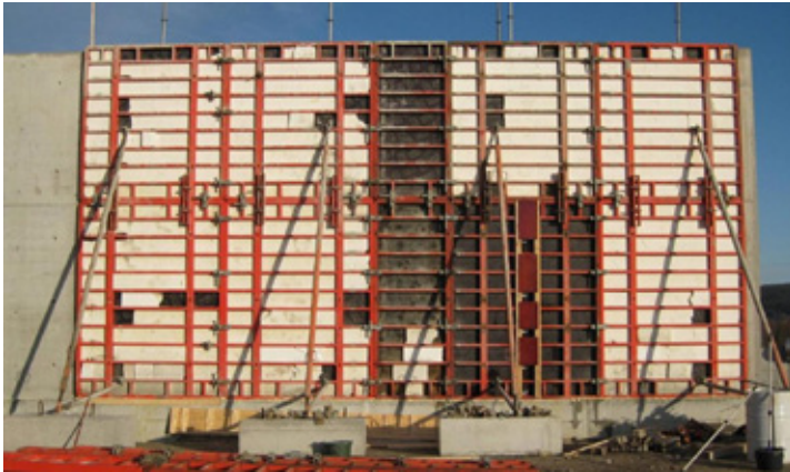
Figure 5 – Location of the instrumented form element in the actual section.
