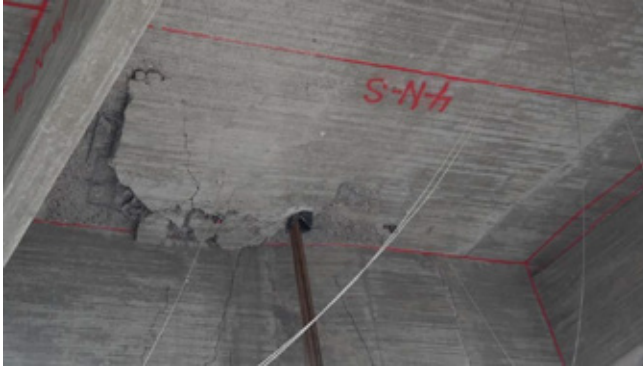
Figure 17 – Photograph of the bridge slab failure, view from south (2014-06-27).
