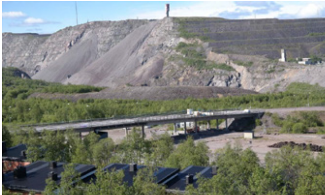
Figure 1 – Photograph of the Kiruna Bridge from the north-east, showing the slag heap from the LKAB iron ore mine in the background (2014-06-25).
