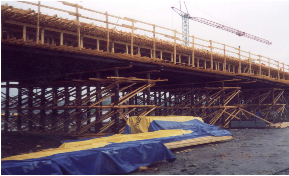
Figure 1. One of the reasons why developments are needed – a common sight from a Swedish bridge construction site today.
