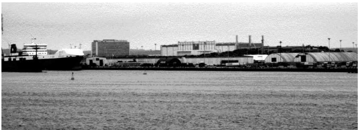
Figure 2A. Overview of wharves
