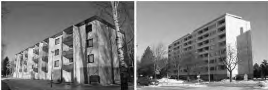
Figure 5 Typical Finnish suburban precast concrete buildings.
