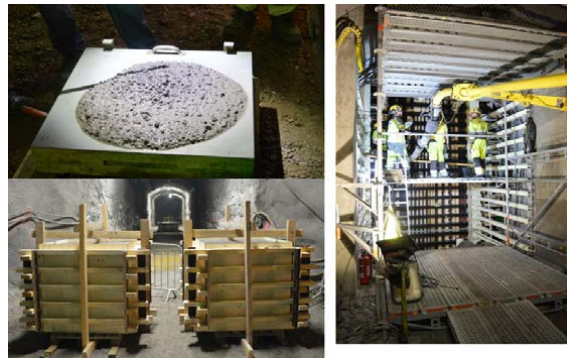
Figure 2 - Casting demo structure underground.
