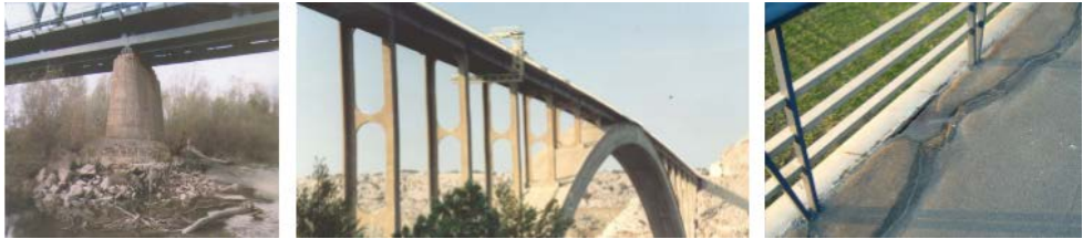
Figure 2 - Three main sub-systems: substructure, superstructure and roadway/equipment, [3].
