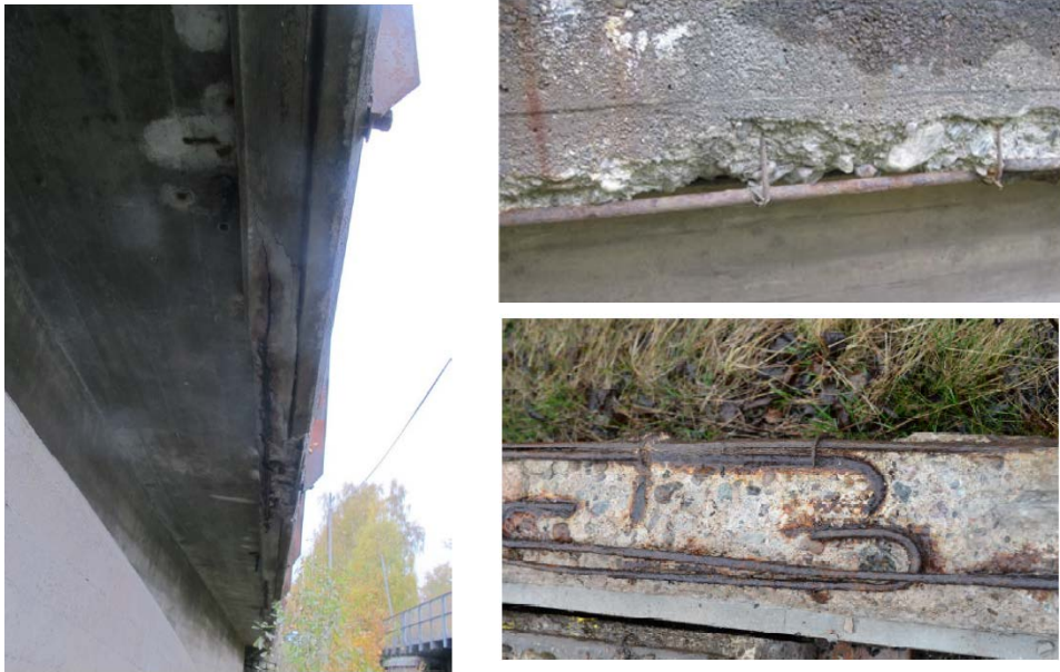
Figure 1 – On the left, the bridge in Gullspång before removal, photo from below showing the bottom side of the edge beam. On the right, a close-up of an edge beam and one of the edge beams after removal, note the hooks.
