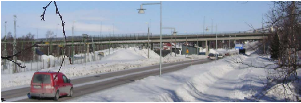
Figure 1. The Kiruna Bridge with road E10 to the right and Iron Ore Railway line to the left (2010-03-23).
