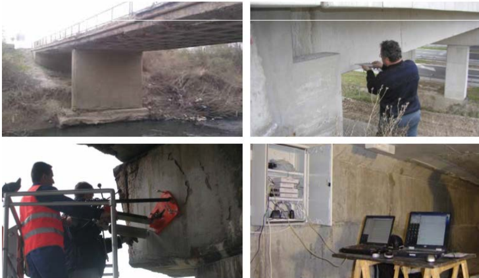
Figure 3 - Main approaches in damage detection: visual inspection, non-destructive testing, probing and structural health monitoring (SHM), [3].
