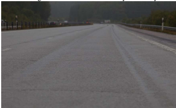
Figure 1 A concrete pavement with rutting in Sweden. Photograph: Fredrik Hellman.
