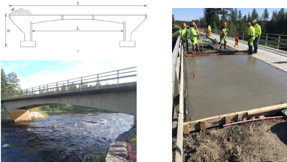
Fig 1. Studied bridge with a span of 25 m and a total length of 37.5 m, bridge deck width: 6.9 m. Concrete overlay casting of one traffic lane.
