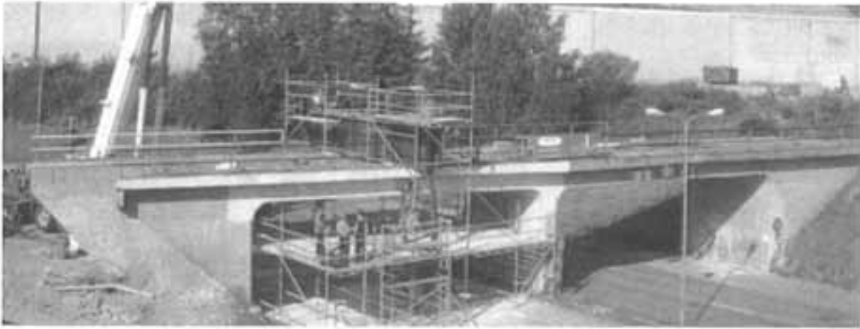
Figure 1 – View of bridge in Örnköldsvik during testing.
