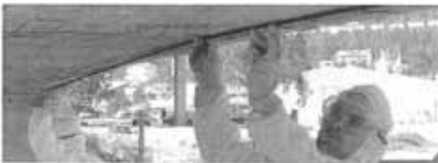
Figure 1 – NSMR strengthening of a railway bridge. Figure 2 – Carbon fibre grid.
