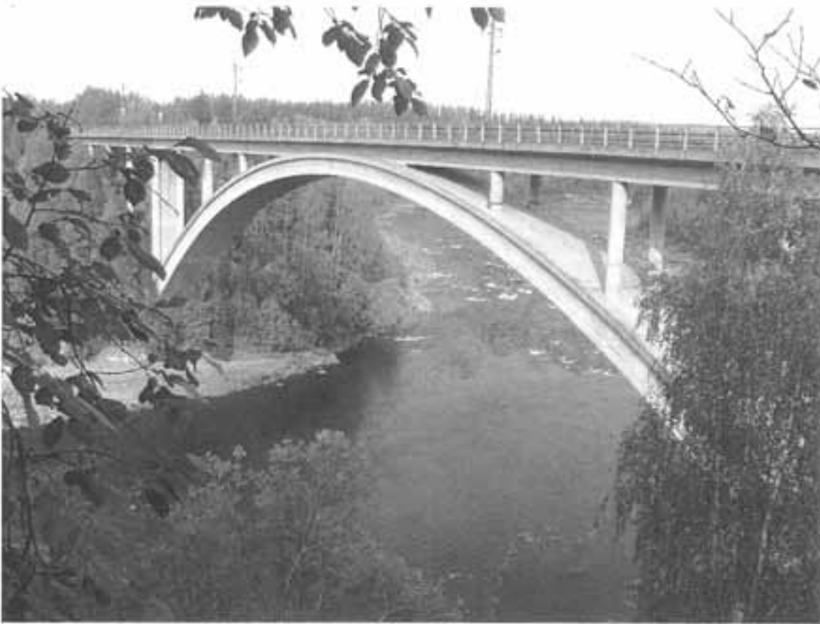
Figure 1 – In order to increase the allowable train axle loads from 22,5 to 25 kN the Vindel Bridge has been assessed with methods developed in the Sustainable Bridges project. The bridge is situated along the Swedish main northern railway line and crosses the Vindel River near Vindeln some 60 km NW of Umeå. It is a concrete arch bridge with a span of 110 m and a height of 22 m, which was constructed in 1952.
