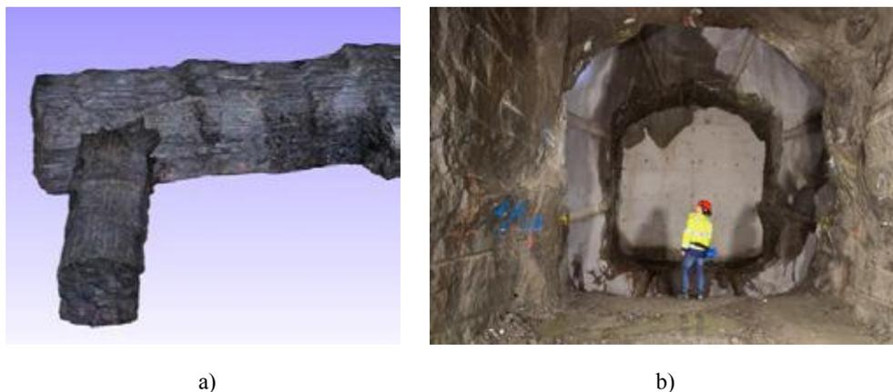
Figure 3 – a) Illustration of the excavated test tunnel based on laser scanning, b) Photo of the excavated slot, in the photo the project leader Pär Grahm (SKB) is shown.
