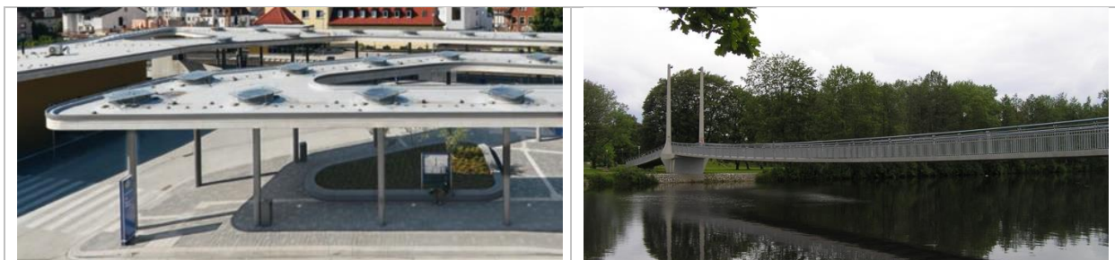
Figure 2 – Left: Bus station roof, Korbach, Germany. Right: Pedestrian bridge Budweis, Czech Republic
