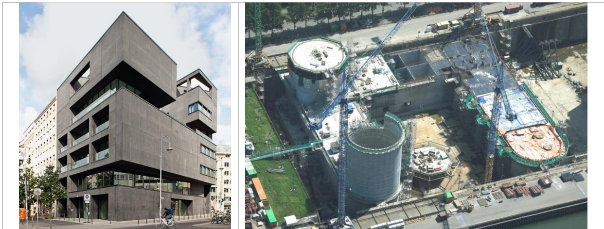
Figure 4 – Left: Linienstraße 40, Berlin, Germany. Right: Heavy lifter, Rotterdam, The Netherlands
