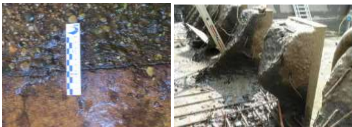
Figure 1 – Abrasion erosion damage of different degree
