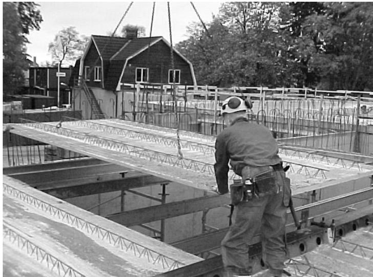
*Figure 1. Mounting of lattice girder elements on the construction site (photo, Hans Olsson SKANSKA, Mellerud).*
