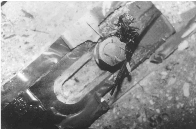
Figure 2 - Shear failure of CFRP laminate.
