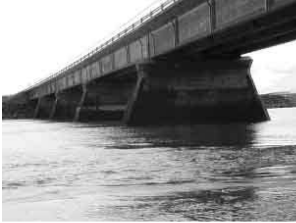
Figure 2. Borgarfjordur bridge. Two piers on the picture have been repaired with cover-concrete. The second one was done with SCC in 2002.
