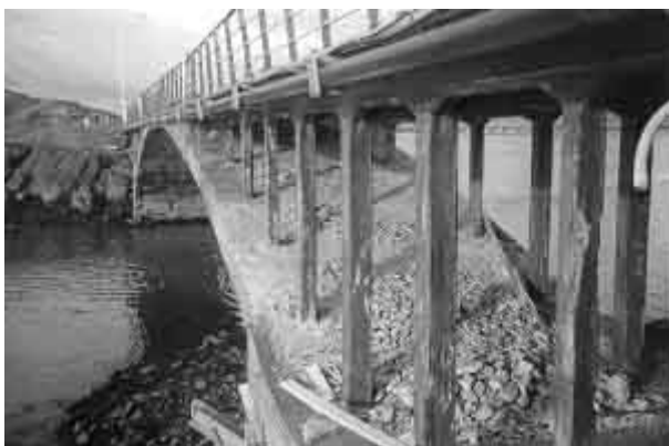
Figure 1. Brakarsund. The picture is taken prior to the repair in 1998. SCC was cast in 2002 in the foundation of the bridge on the near end of the bridge where the wooden moulds are. The picture is taken at low tides. The foundations were submerged in sea water within two hours.
