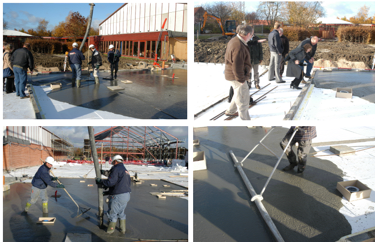
Figure 6 - Pictures from the excursion to a job site in Ishøj, Denmark [Pictures taken by Kjell Wallin].
