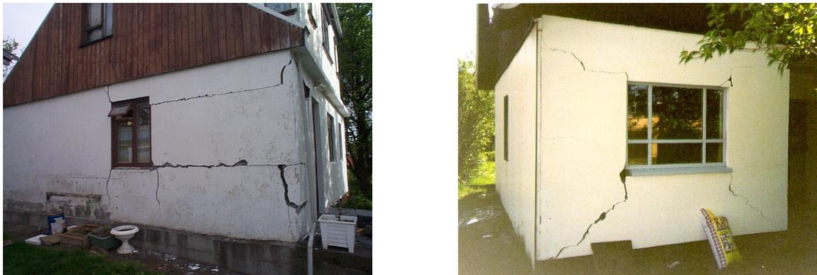
*Figure 1 - Houses damaged during the South Iceland earthquakes of June 2000.*
